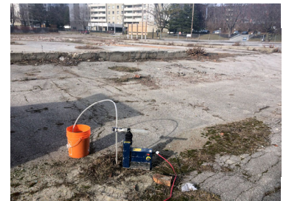
Fig. 2—Developing a monitoring well at the Site
