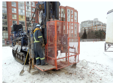
Fig. 1—Drilling to investigate soil and groundwater quality at the Site
