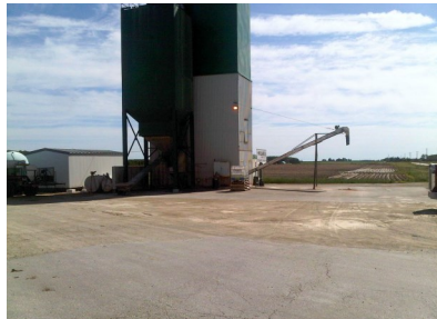
Fig. 1—On-site fertilizer processing plant
